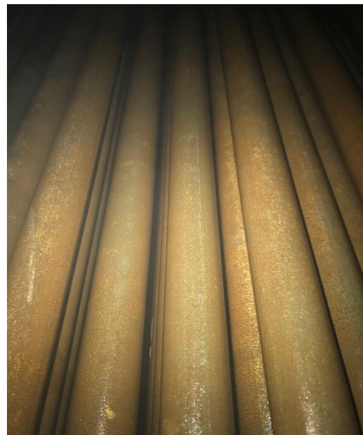
Scaled boiler tubes before cleaning boiler tubes after chemical clean
